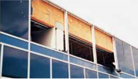
This glass wall facade was destroyed by high winds, leaving the building interior vulnerable to wind and rain damage.
