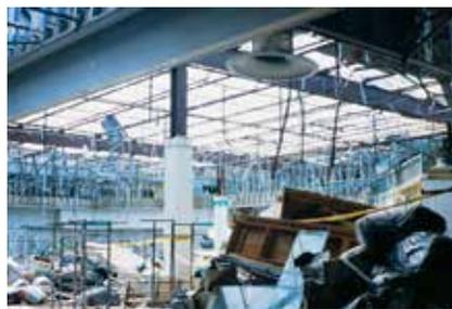
An insulated steel-deck roof was blown off this building.
