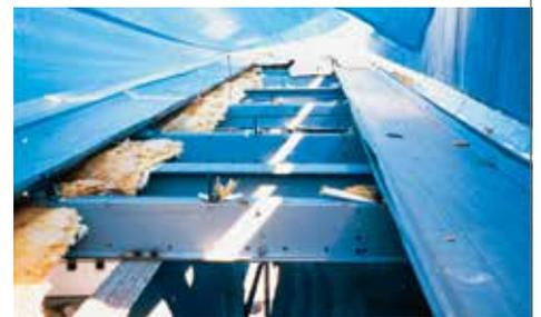
Panels of this standing-seam deck were torn off; leaving the fasteners still attached to the roof framing.
