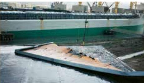
The damaged roof covering on this seaport building is mostly along the edge where wind forces are at a maximum.
