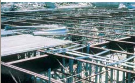
The lightweight concrete on this metal roof was severely damaged by a tropical storm.
